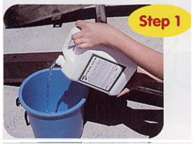
Clean the rust or corroded metal with Marine Clean, an environmentally safe cleaner. Marine Clean will remove dirt, grease, wax or other contaminants that could interfere with the restoration. Rinse off with water.
